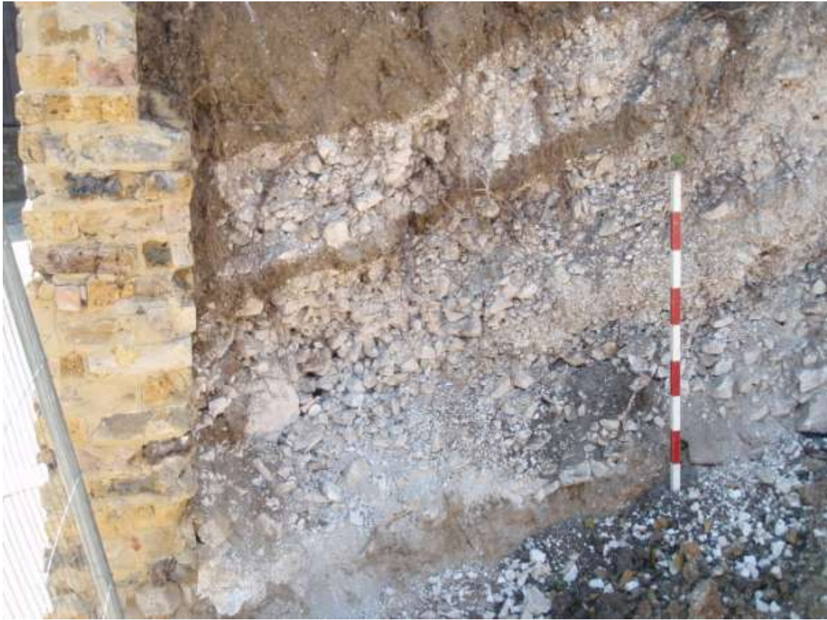
Plate 4. Excavation for access for car park bay to Castle View Road showing made-up ground (facing east)
